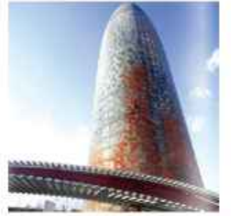
Torre Agbar, Barcelona, Spain
