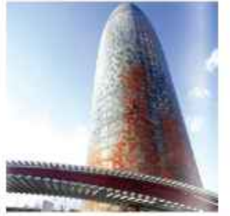
Torre Agbar, Barcelona, Spain
